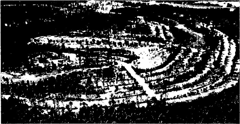
This photo shows the development of a tract of ground where the builder is making good use of the natural topography and preserving part of the natural tree cover.
