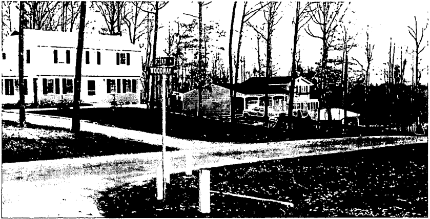
Conservation at building sites is demonstrated by this project where trees and other vegetation have been spared and construction has followed the natural contours of the land. Note well-shaped road drain protected by grass in right foreground.
